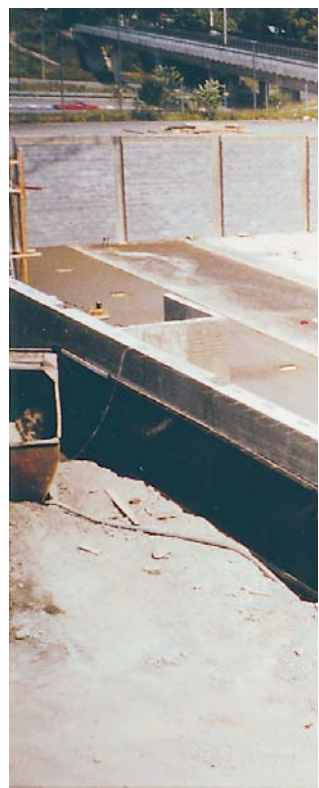
Underetasjen tar form.
